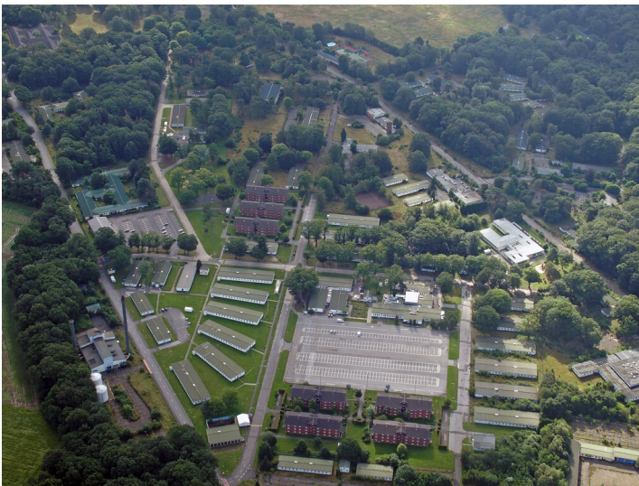
Joint Headquarters JHQ Rheindahlen in Mönchengladbach (2021) Fotograf/Urheber: Karl Peter Wiemer
